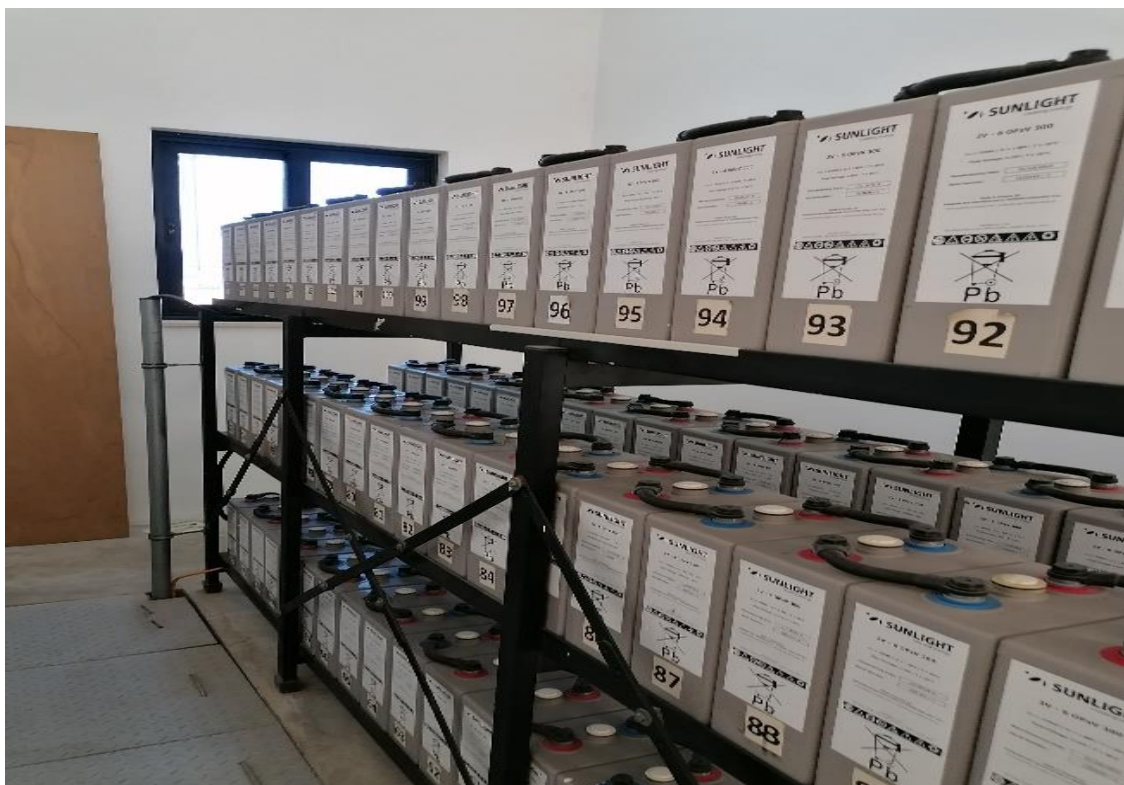
Picture (10): UPS system batteries
