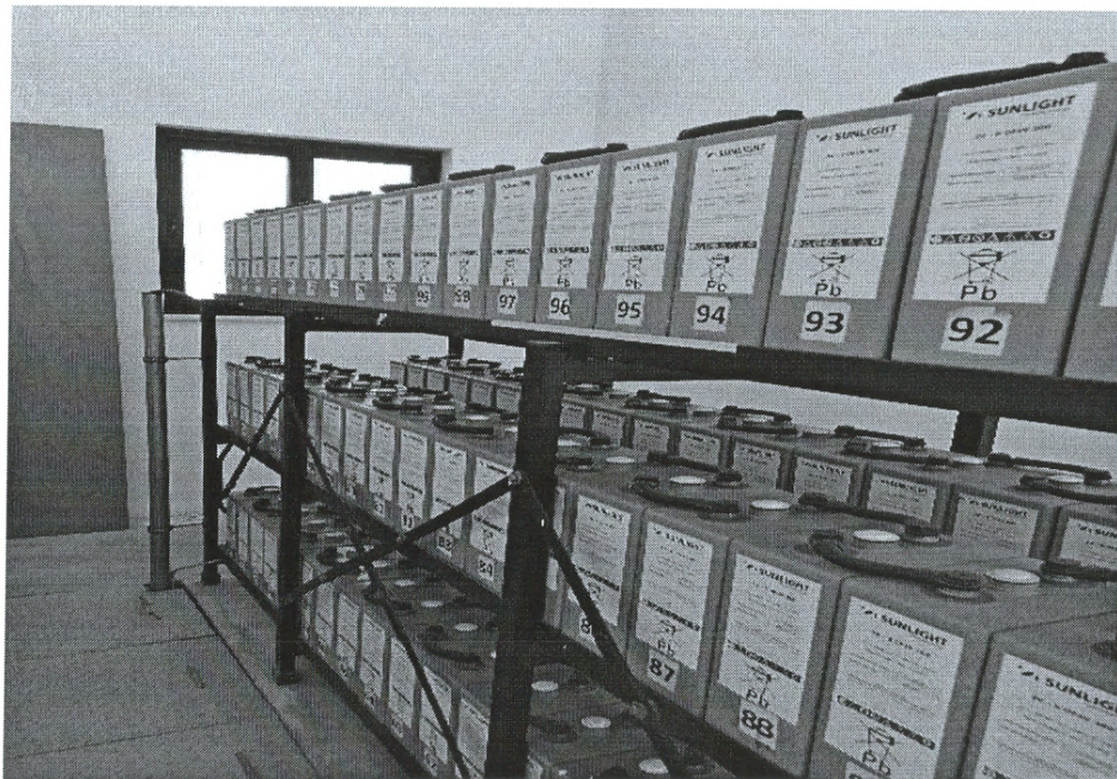
Picture (10): UPS system batteries
