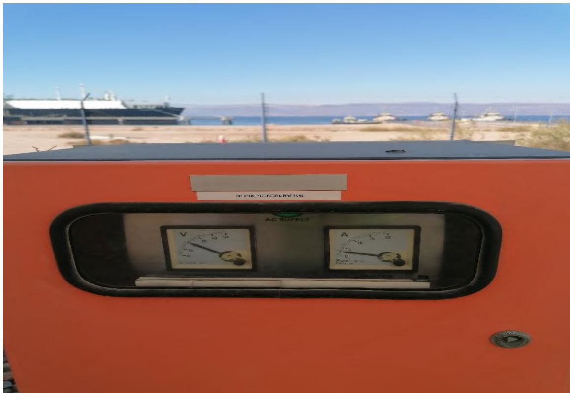
Picture (12): Cathodic protection system main supply
